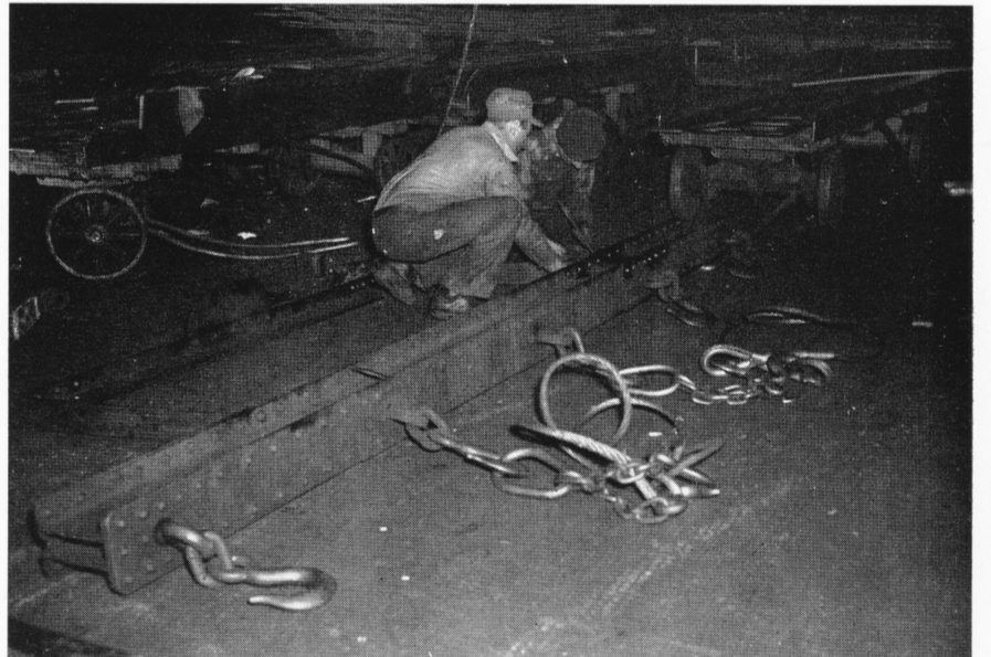
Like all other machinery, cranes need constant attention. The boom uprights have become bent here, and Hank and Johnny are putting in new ones. If the Electrical Department can't straighten them, they are sent to the Blacksmith shop. With all the precautions, never walk under suspended loads.
